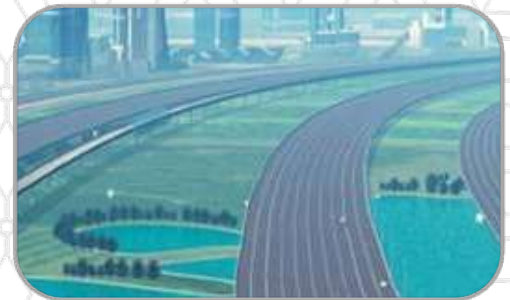
250 M WIDE 10 LANE AHMEDABAD - DHOLERA EXPRESS WAY
