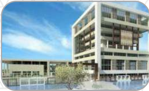
DHOLERA ABCD BUILDING
