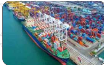
Port And Cargo Terminal
