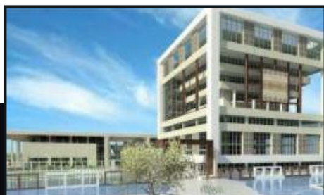
DHOLERA ABCD BUILDING
