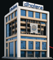
Dholera ABCD Building
