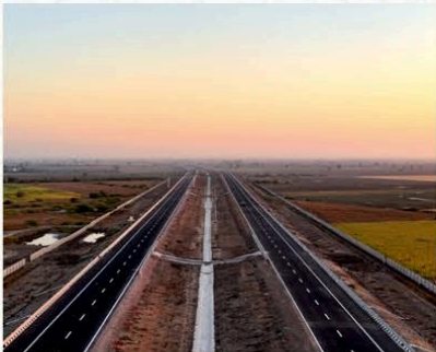
Dholera Expressway 109 km long expressway project. 4-lane access-controlled highway for fast travel. Links Ahmedabad to Dholera Smart City directly.
