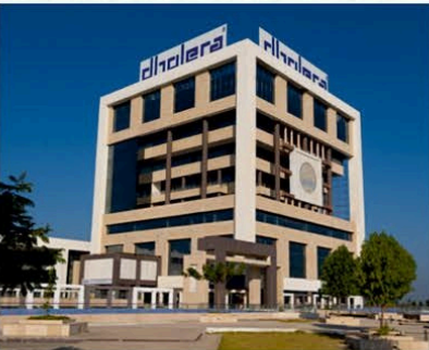
ABCD Building Administrative building with city Integrated Operation Center
